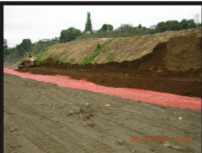
Photo 20 Haul road of clean topsoil being spread over demarcation fabric.
