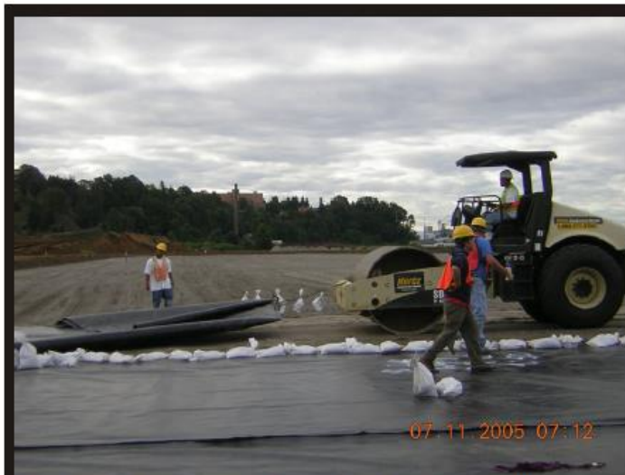
Photo 23 Geomembrane being deployed utilizing a roller.
