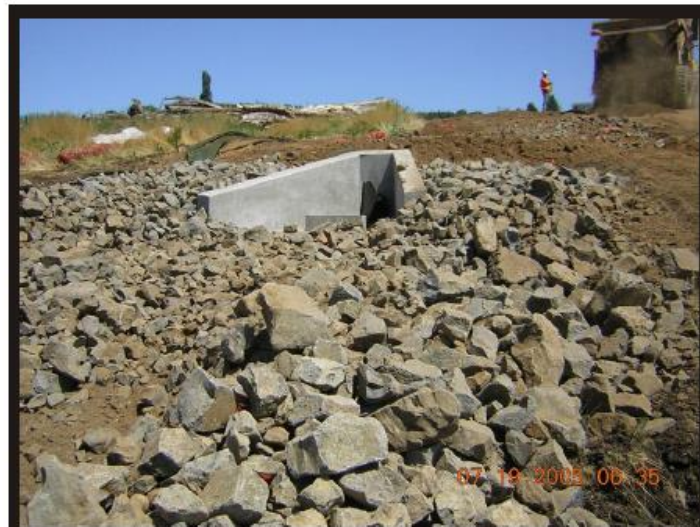
Photo 14 Outfall structure and 12" minus rock below the outfall.
