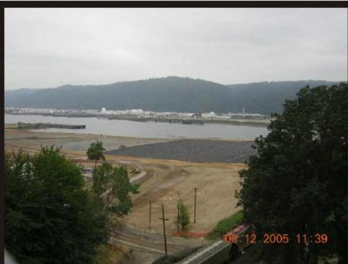
Photo 36 Overview of site showing biotic rock layer and overlying geotextile layer.
