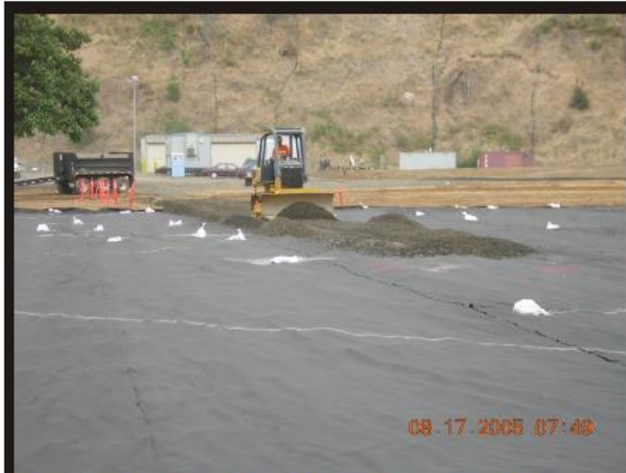
Photo 37 Placement of gravel for access road across the impermeable cap.
