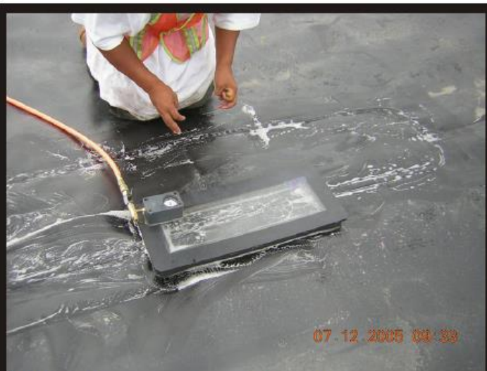
Photo 28 Vacuum testing geomembrane patch.
