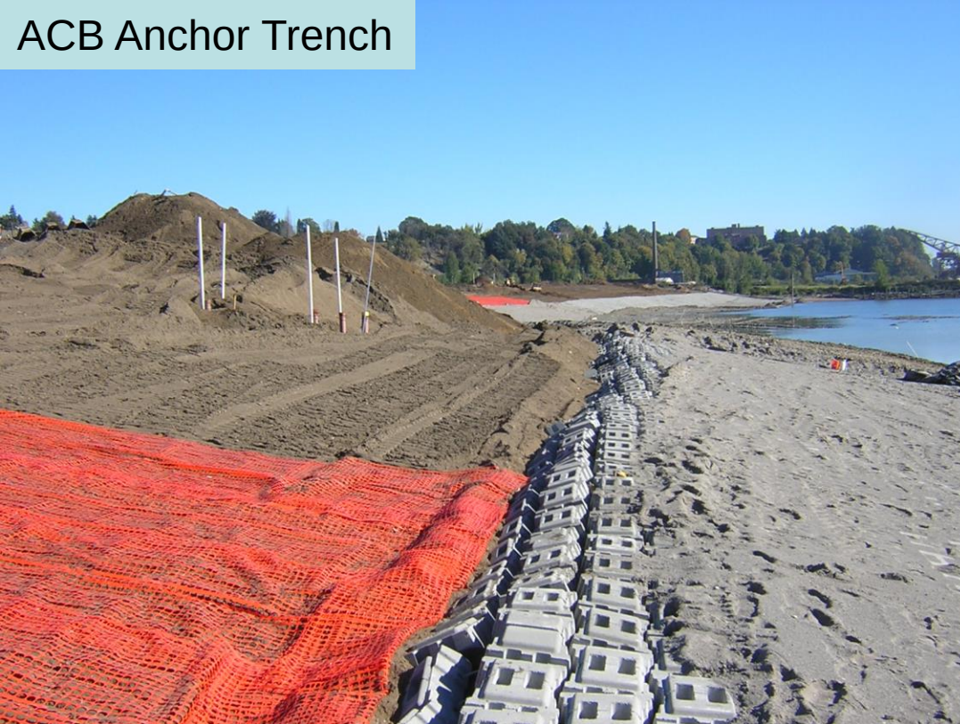
Bank Stabilization and Capping (2004)
