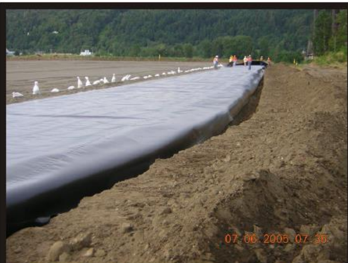
Photo 22 First panel of geomembrane being installed along the north end of the impermeable cap footprint.
