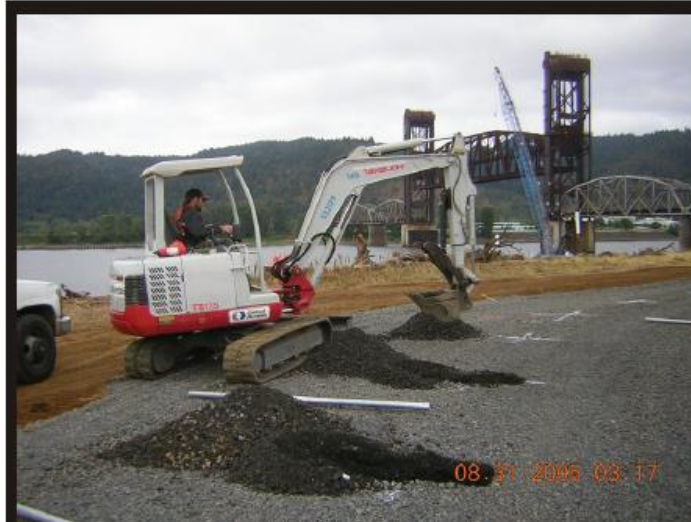
Photo 45 Willamette Fence Co. digging post holes.
