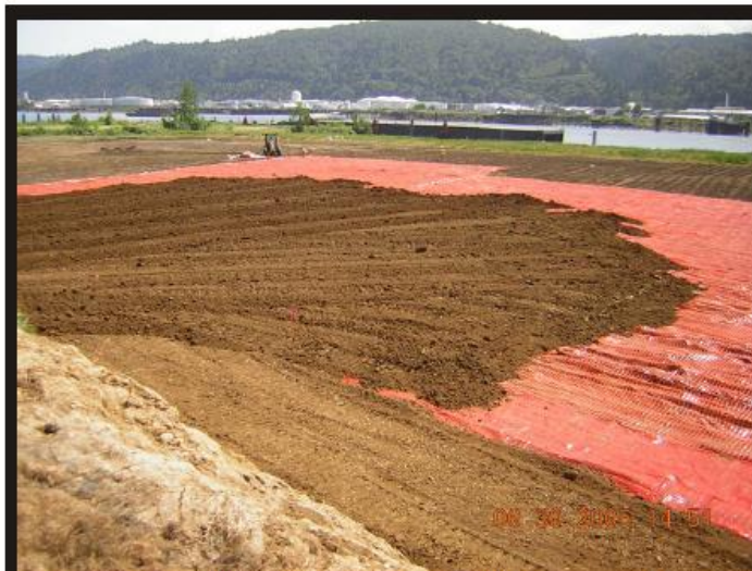
Photo 21 Topsoil from the existing stockpile being spread out over demarcation fabric.
