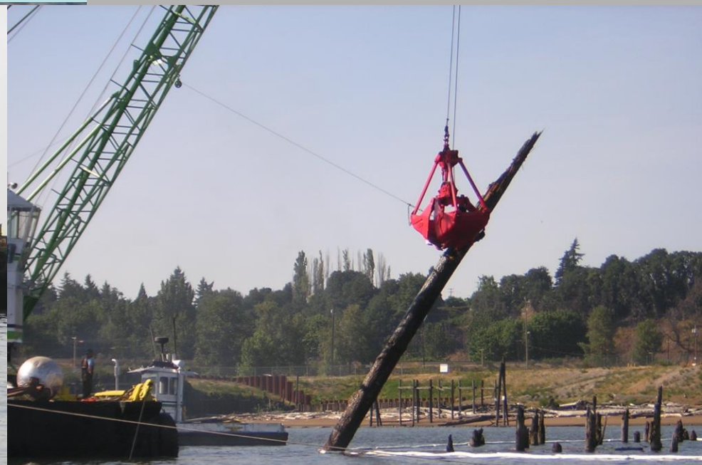
Pulling Additional Pilings (ESA Mitigation)
