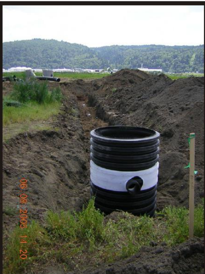
Photo 8 Manhole D with a partially installed pipe to Manhole E.
