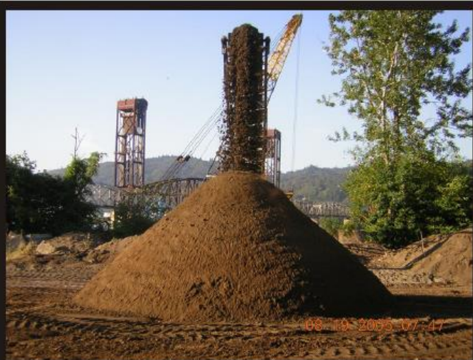
Photo 38 Topsoil unloaded from barge with conveyor.
