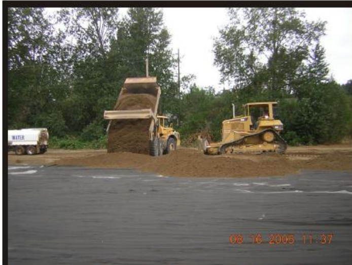
Photo 39 Topsoil being placed over geotextile within the impermeable cap footprint.
