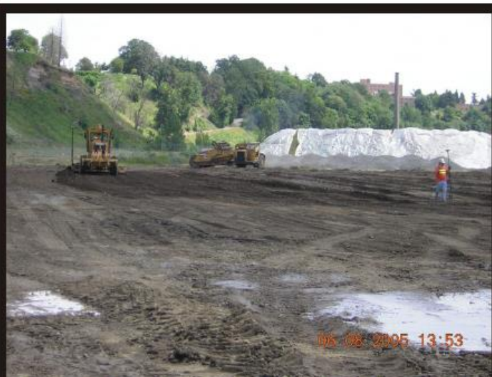
Photo 1 Subgrade preparation along eastern edge of property.
