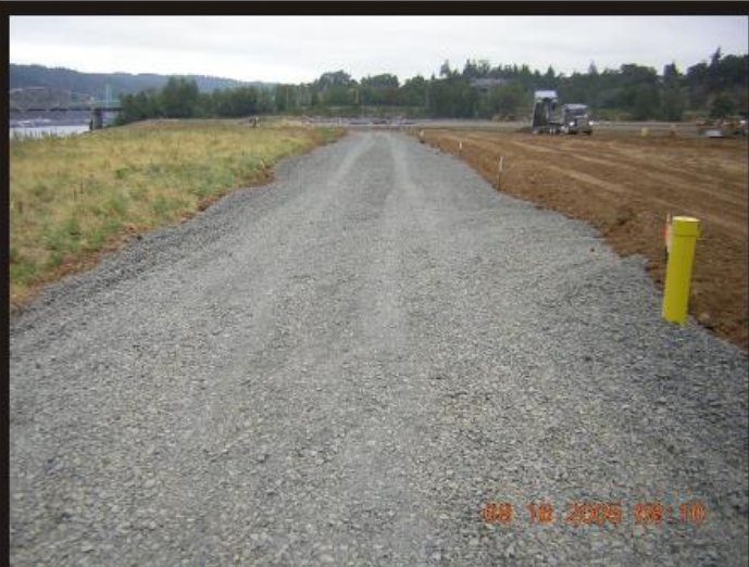
Photo 44 Gravel road along top of the bank.
