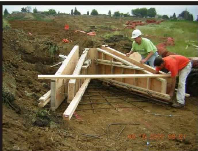
Photo 13 Form for concrete outfall structure being constructed.
