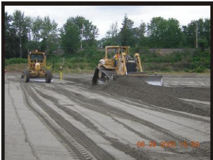
Photo 18 Placing the leveling sand layer.
