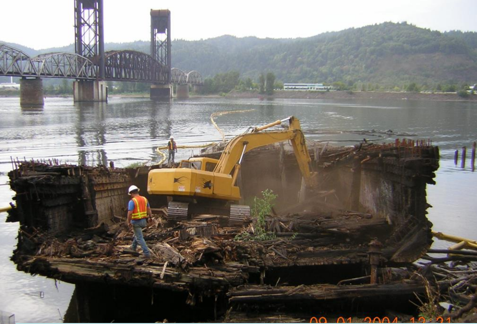
Derelict Barge Demolition (ESA Mitigation)
