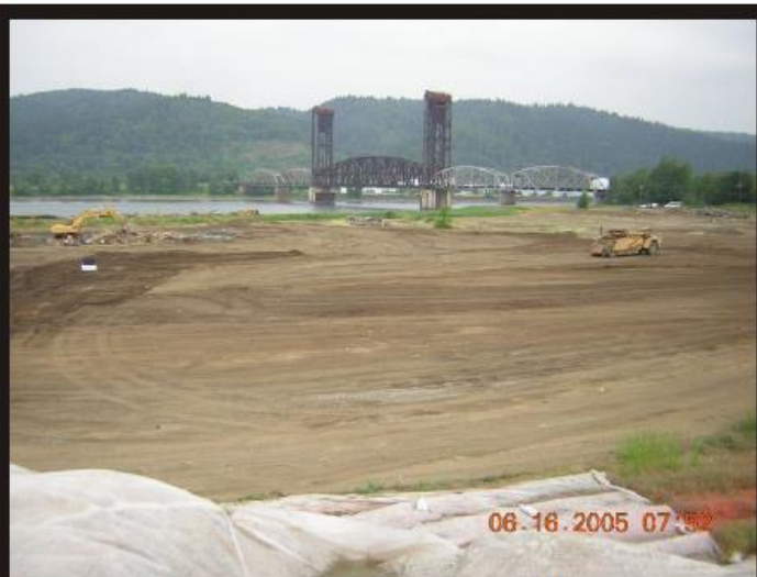
Photo 3 Subgrade activities for the impermeable cap.
