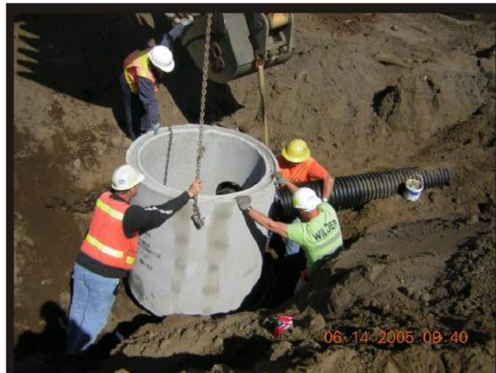
Photo 12 Installation of Manhole E.
