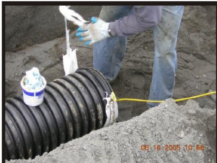
Photo 9 Applying grease to the ends of conveyance piping prior to coupling.
