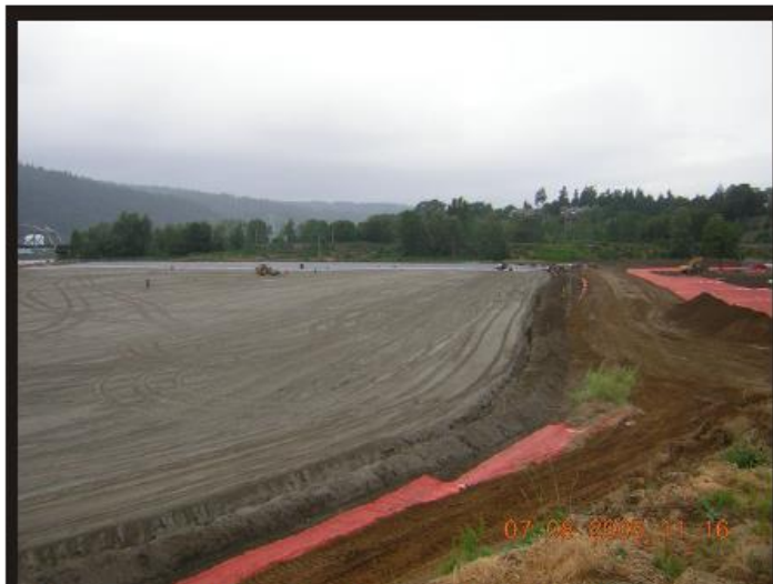
Photo 29 Overview of site with completed leveling layer and partial installation of geomembrane.
