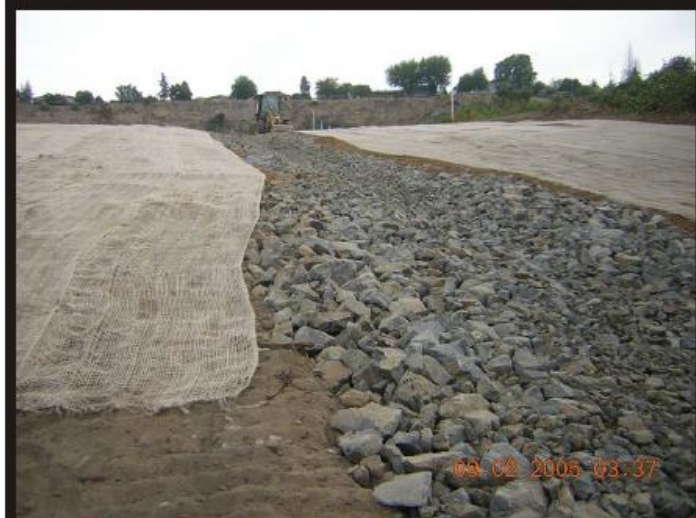
Photo 43 Erosion control netting installed around pond spillway.
