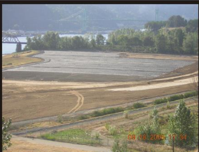
Photo 40 Overview of site showing three layers of impermeable cap. Starting from the foreground: 4" minus biotic rock, geotextile, and topsoil.
