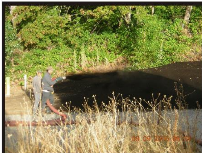
Photo 50 Applying compost prior to hydroseeding on bank areas disturbed during construction.
