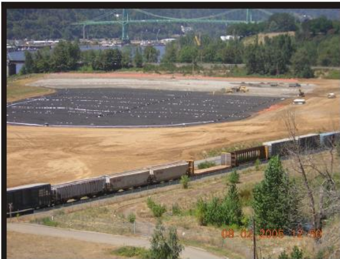
Photo 35 Overview of site showing three layers of impermeable cap. Starting from the foreground: geocomposite layer, drainage sand layer, and 4" minus biotic rock layer.
