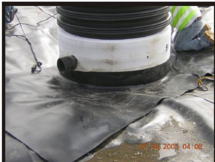
Photo 25 Installation of boot around Manhole B.
