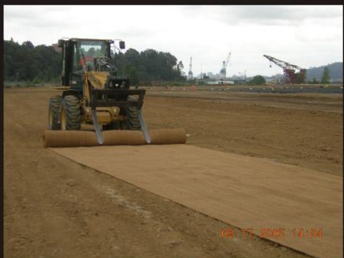
Photo 42 Deploying erosion control netting along the swale area.
