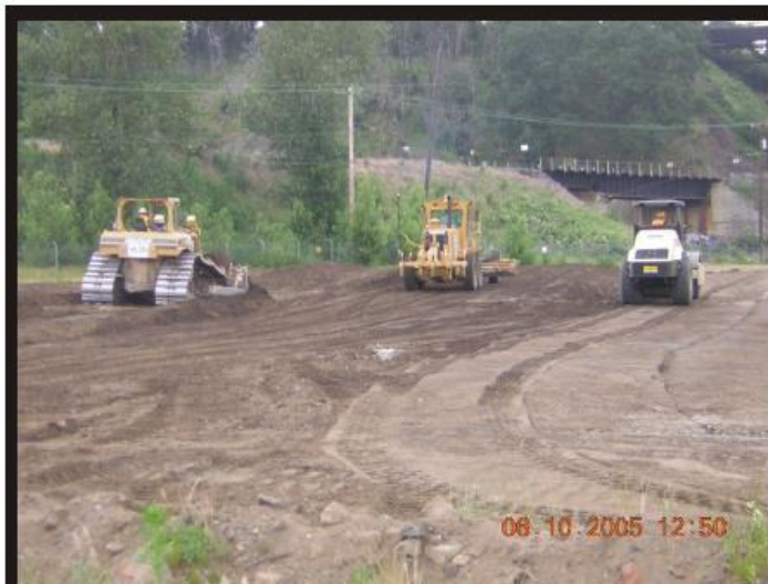
Photo 2 Subgrade grading and cut/fill near NE corner of property.
