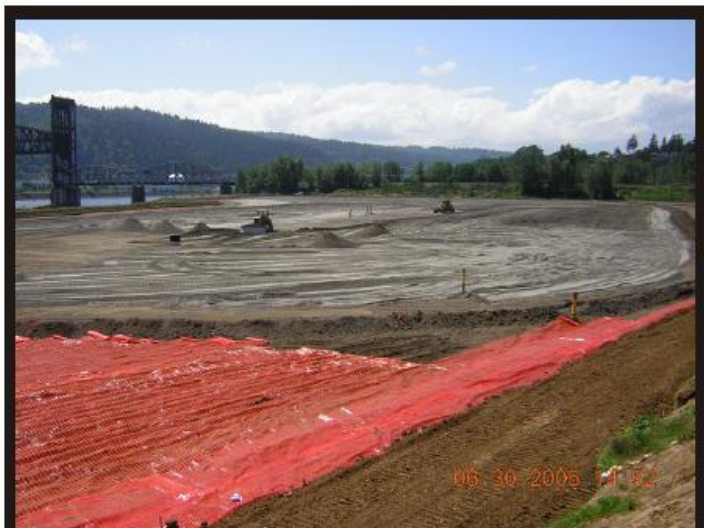
Photo 19 Rough placement of sand leveling layer nearly completed.
