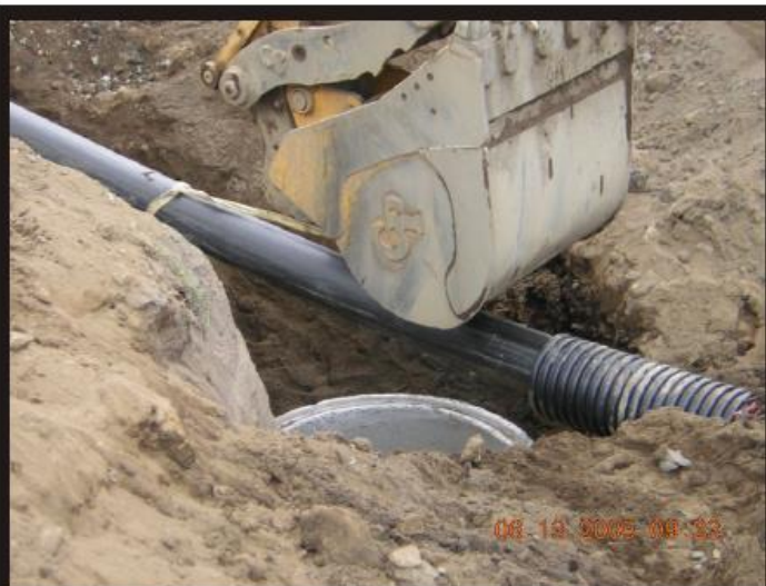
Photo 11 Excavator used to slide the smooth wall interior conveyance piping into the outer corrugated piping.
