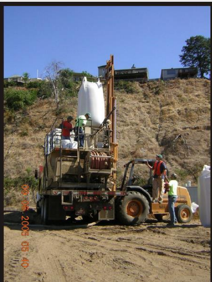
Photo 48 Placing mineral supplements into hydroseeding mixing tank.
