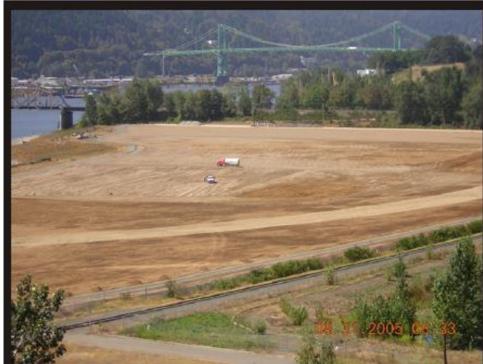
Photo 41 Topsoil placement complete over the impermeable cap footprint.
