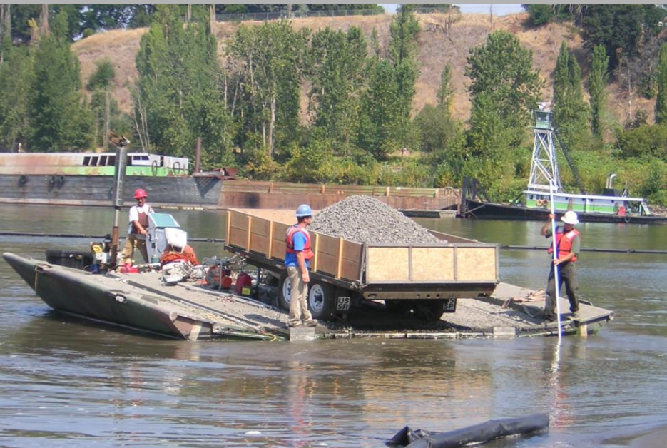
Rock Armoring Placement
