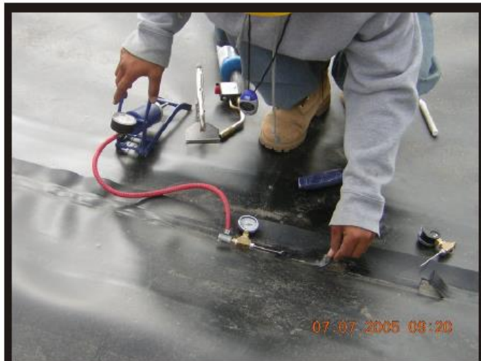
Photo 27 Air pressure testing geomembrane seam.
