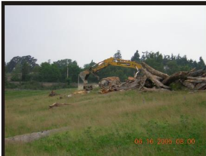
Photo 4 Placement of large woody debris along the top of bank.
