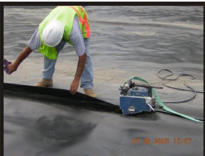
Photo 24 Welding geomembrane panels with wedge welding machine.
