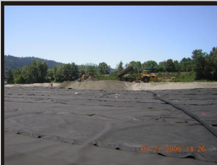
Photo 33 Placement of the drainage sand layer.
