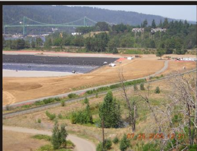
Photo 32 Overview of site showing four layers of impermeable cap. Starting from the foreground: sand leveling layer, geomembrane layer, geocomposite layer, and drainage sand layer.
