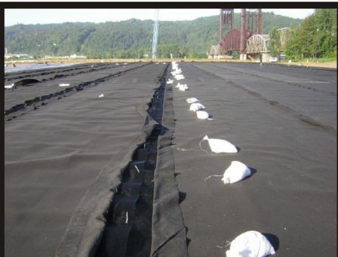
Photo 30 Seams of geocomposite zip-tied together (left), and seams after they've been heat-tacked (right).
