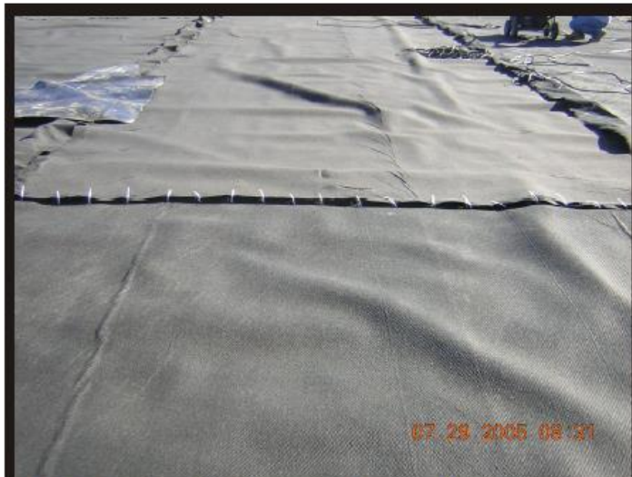
Photo 31 Butt seam of geocomposite zip-tied together.
