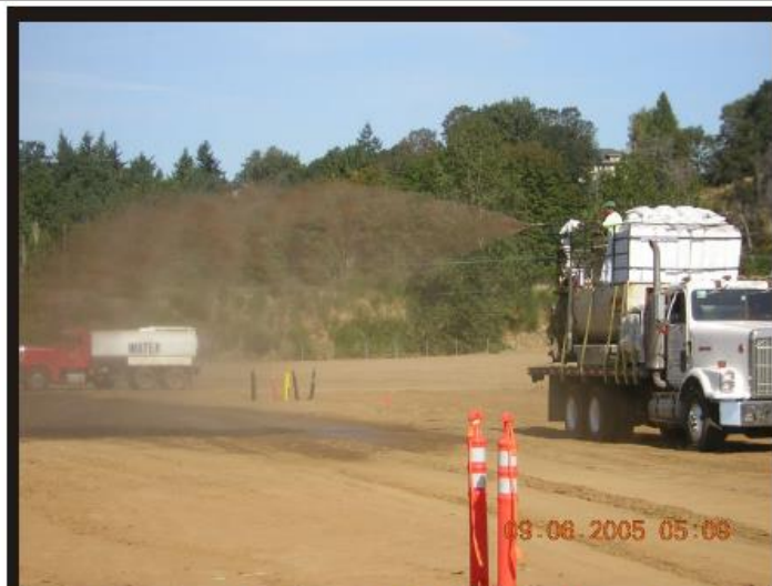
Photo 49 Applying hydroseed on the impermeable cap topsoil.
